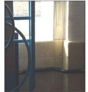
8. Middle hall window sill inside (right front)
