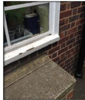
7. Main corridor window sill (right)
